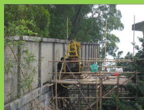
The rig was dismantled into pieces and transported by laborers up to the platform
