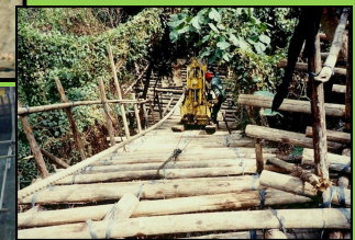
Moving Along Scaffolds by self-winching
